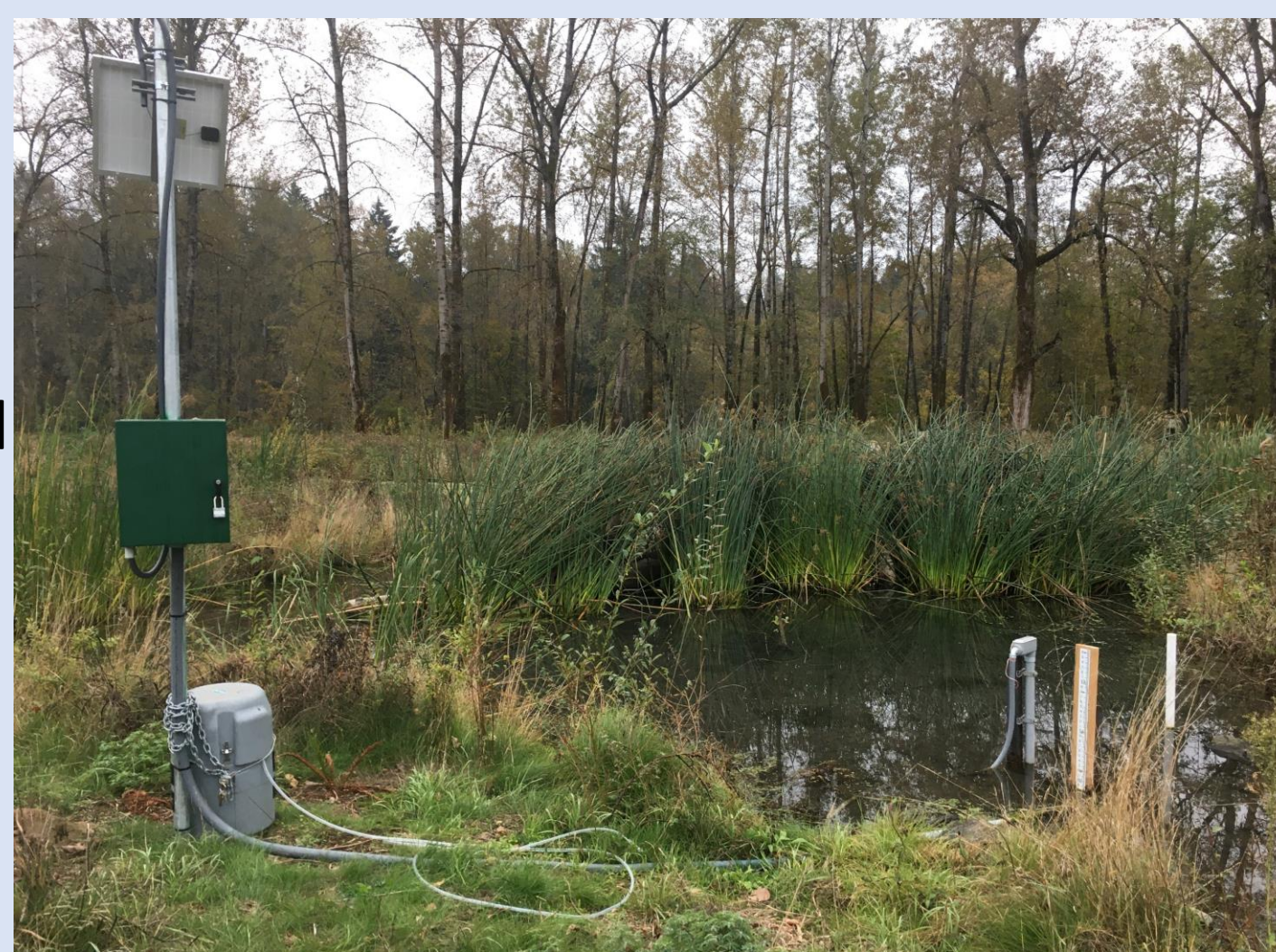
Site 3 showing solar panel, data logger enclosure, sampler, and sensor infrastructure.
